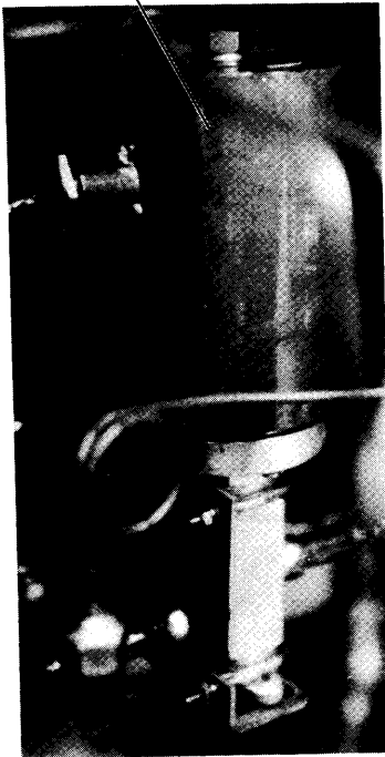
Modulating control valve
